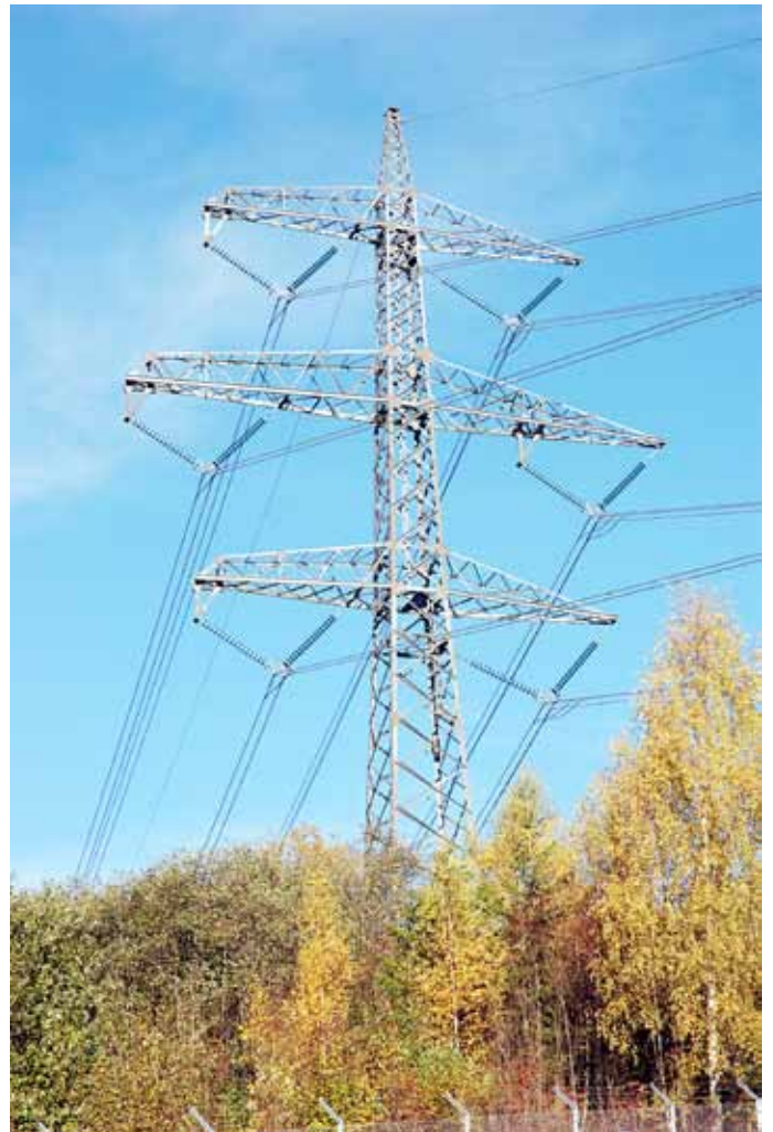
Transmission line 420 kV
